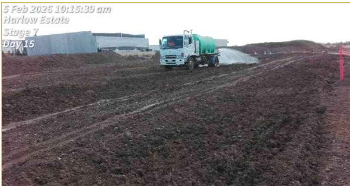
Figure 7: Moisture Conditioning Fill Material (Source: C&T)
