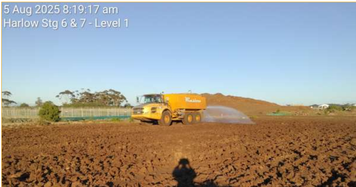
Figure 4: Moisture Conditioning Subgrade Prior to Fill Placement (Source: C&T)
