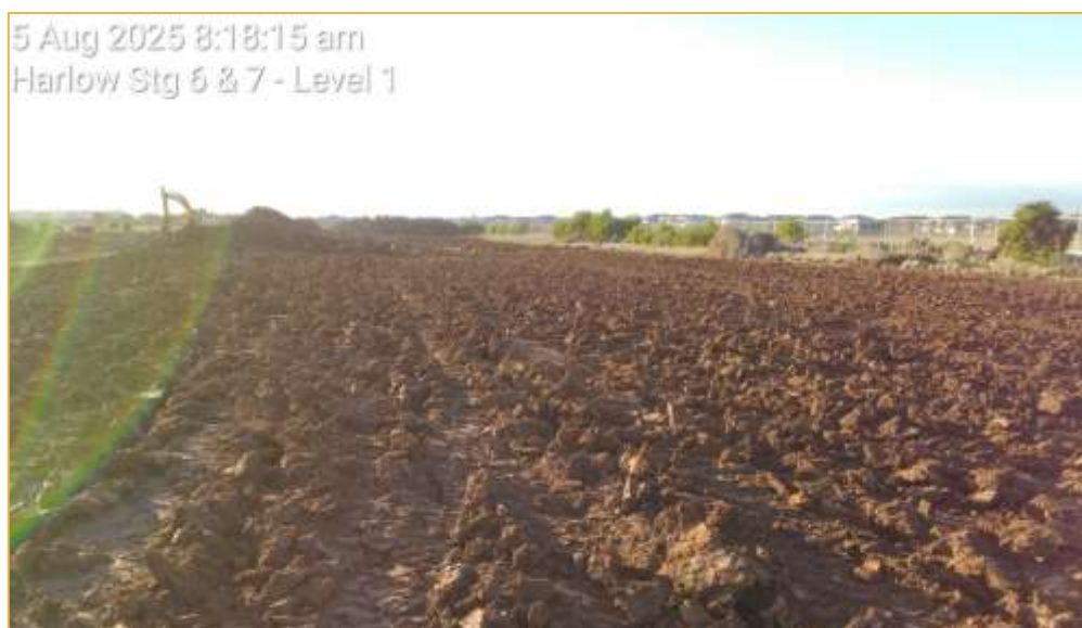
Figure 3: Subgrade Ripped Prior to Fill Placement (Source: C&T)
