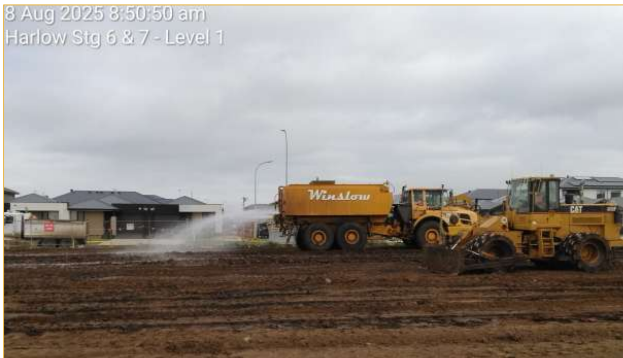
Figure 5: Spreading of Fill Material & Moisture Conditioning (Source: C&T)
